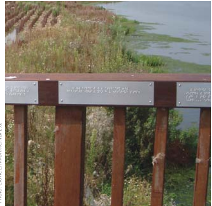
Photo: Crane Environmental Ltd.
