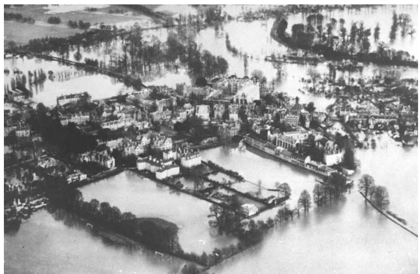
Flooding from the River Thames into Windsor in 1947
