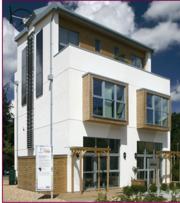
Stewart Milne Group demonstration Sigma Home, on the BRE Innovation Park, achieving 100 per cent reduction in carbon dioxide emissions from heating and lighting.
