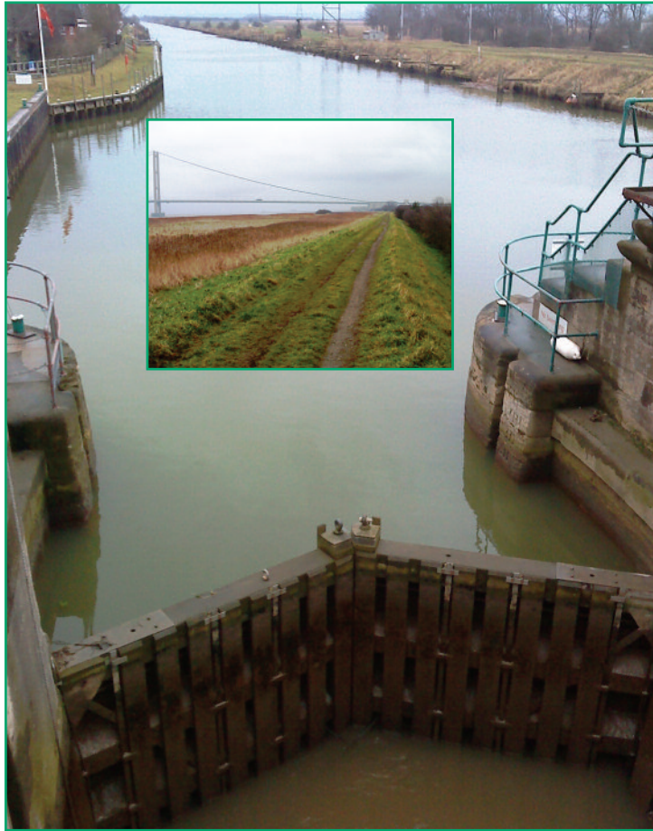
(Inset) Typical Humber Estuary flood defences (Above) Ferriby sluice gate provides key flood protection at the River Ancholme's confluence with the Humber Estuary
