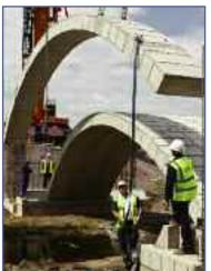
Figure 1 (top): The key elements of the FlexiArch design. Figure 2 (above): Construction of a FlexiArch Bridge.
